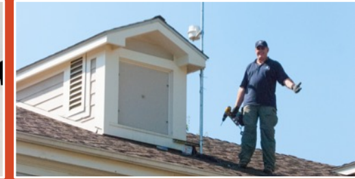
Managed Weather Equipment
