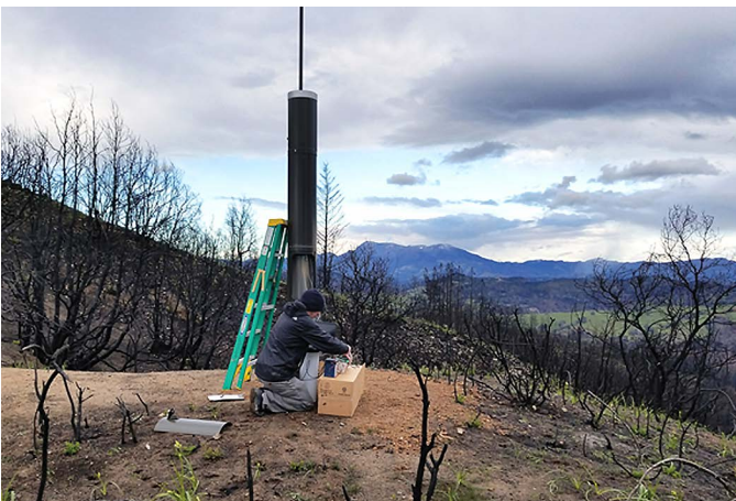
OneRain engineers install new High Sierra Electronics' ALERT2 rain gauge on burn-scarred hillside
