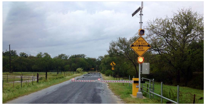
Driver Warning Systems warn motorists via flashers and/or gates of flooded roadways
