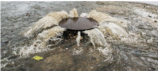
Urban drainage and sewer overflow
